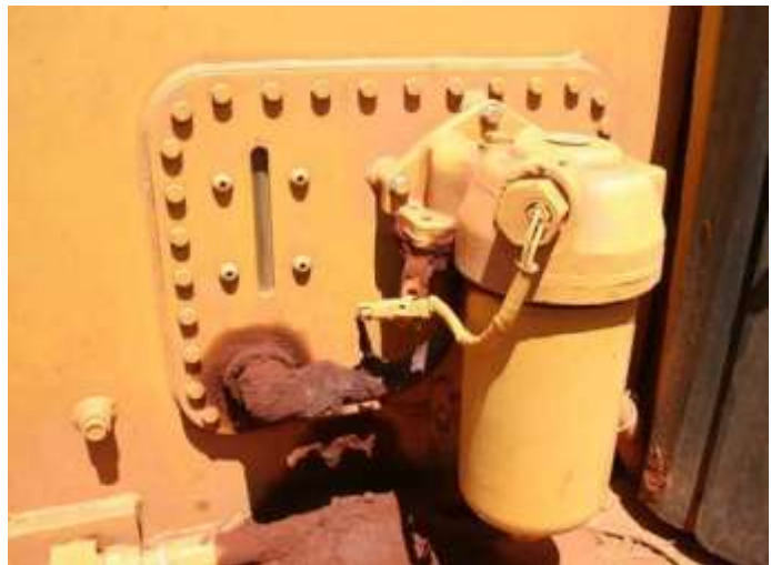
Hydraulic Oil Tank and Sight Gauge
