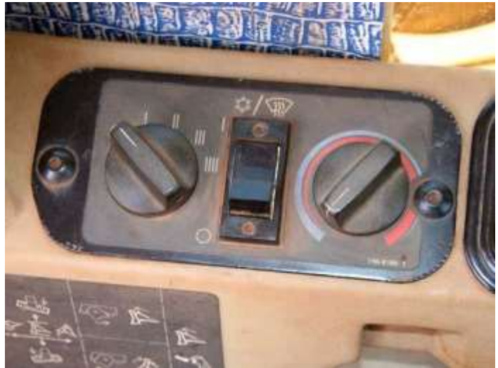
Air Conditioning Controls
